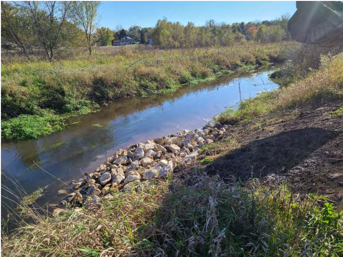
Figure 2: Rock Deflector in Section C of Dane County's Streambank Improvements Project
