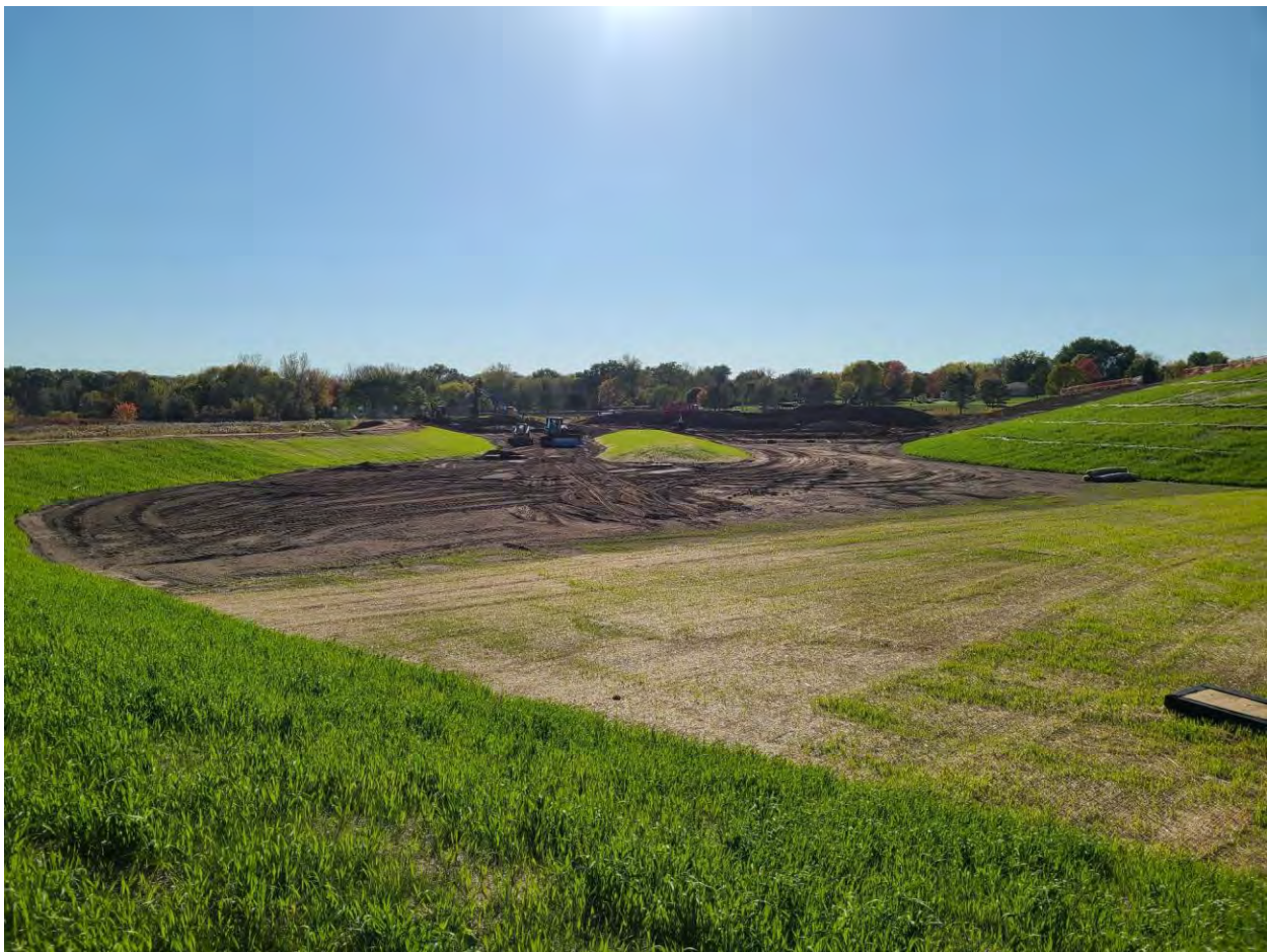
Figure 3: Placement of Remaining Engineered Soil in the Infiltration Pond.
