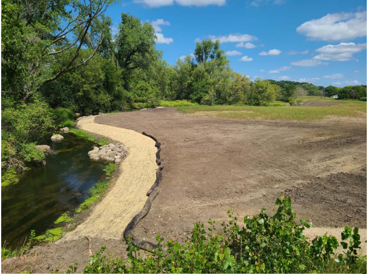
Figure 1: Completed City of Verona Streambank Improvements just north of Bruce Street, with seed restoration beginning.
