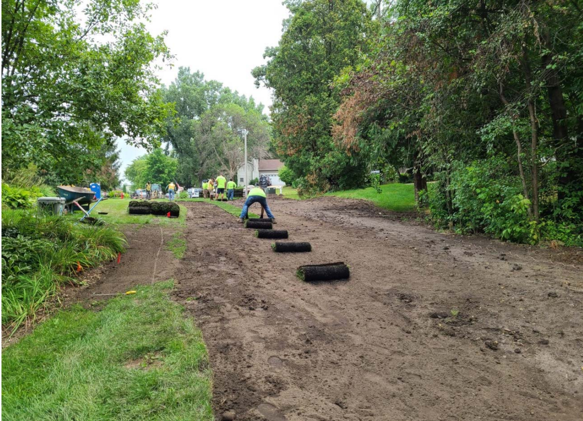
Figure 1: Sod placement at the Arbor Vitae/Local H Connection
