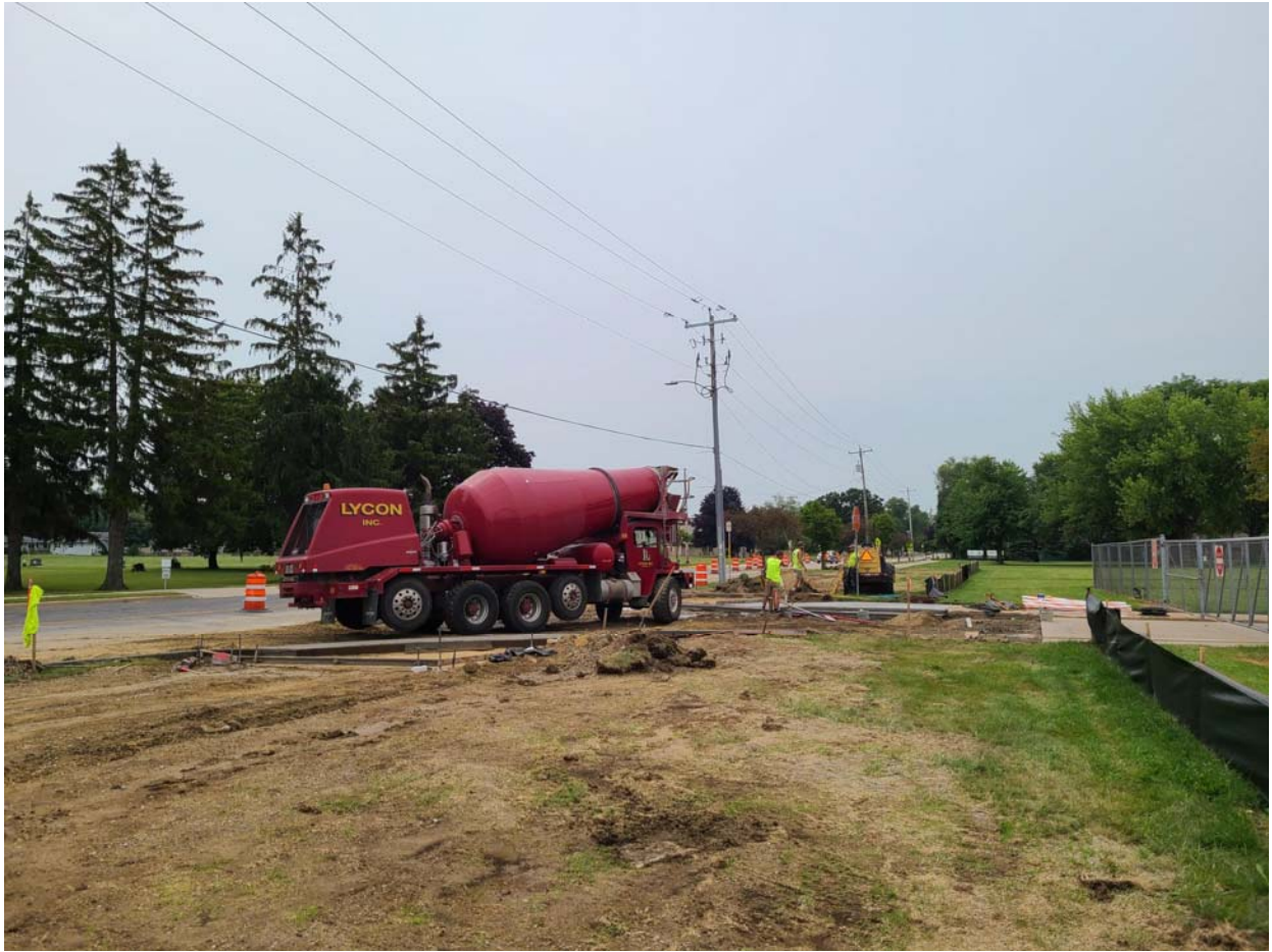
Figure 3: Curb and Gutter and Sidewalk Placement along North Main Street
