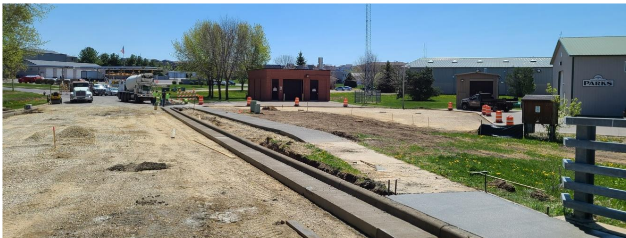
Figure 1: Concrete Curb and Gutter and Sidewalk Along Bruce Street
