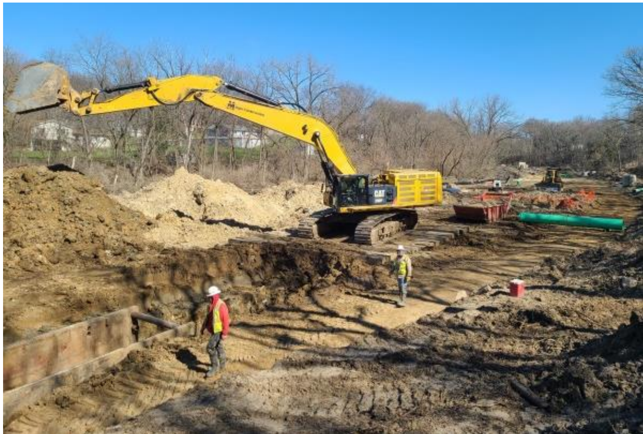
Figure 1: Pipe Operations Moving East Toward Lincoln Street Bridge
