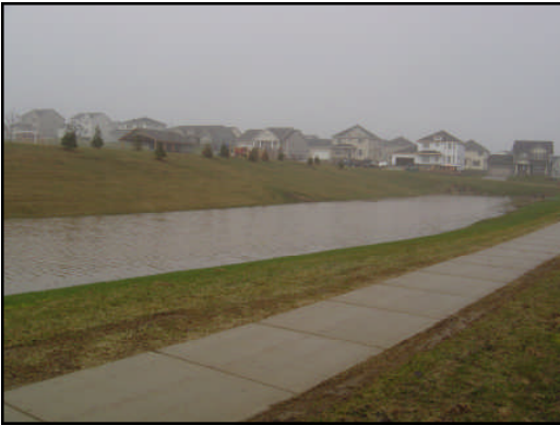
Storm water detention facilities in the City of Verona are designed to prevent flooding, protect local surface waters, and promote ground water recharge.
