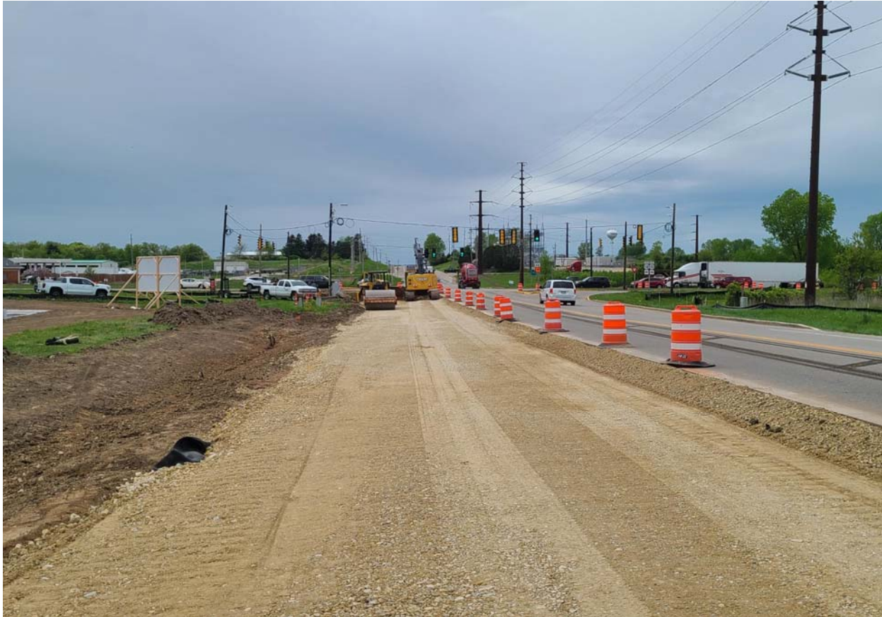
Figure 1: Stage 2 Widening on EB CTH M, East of the Intersection
