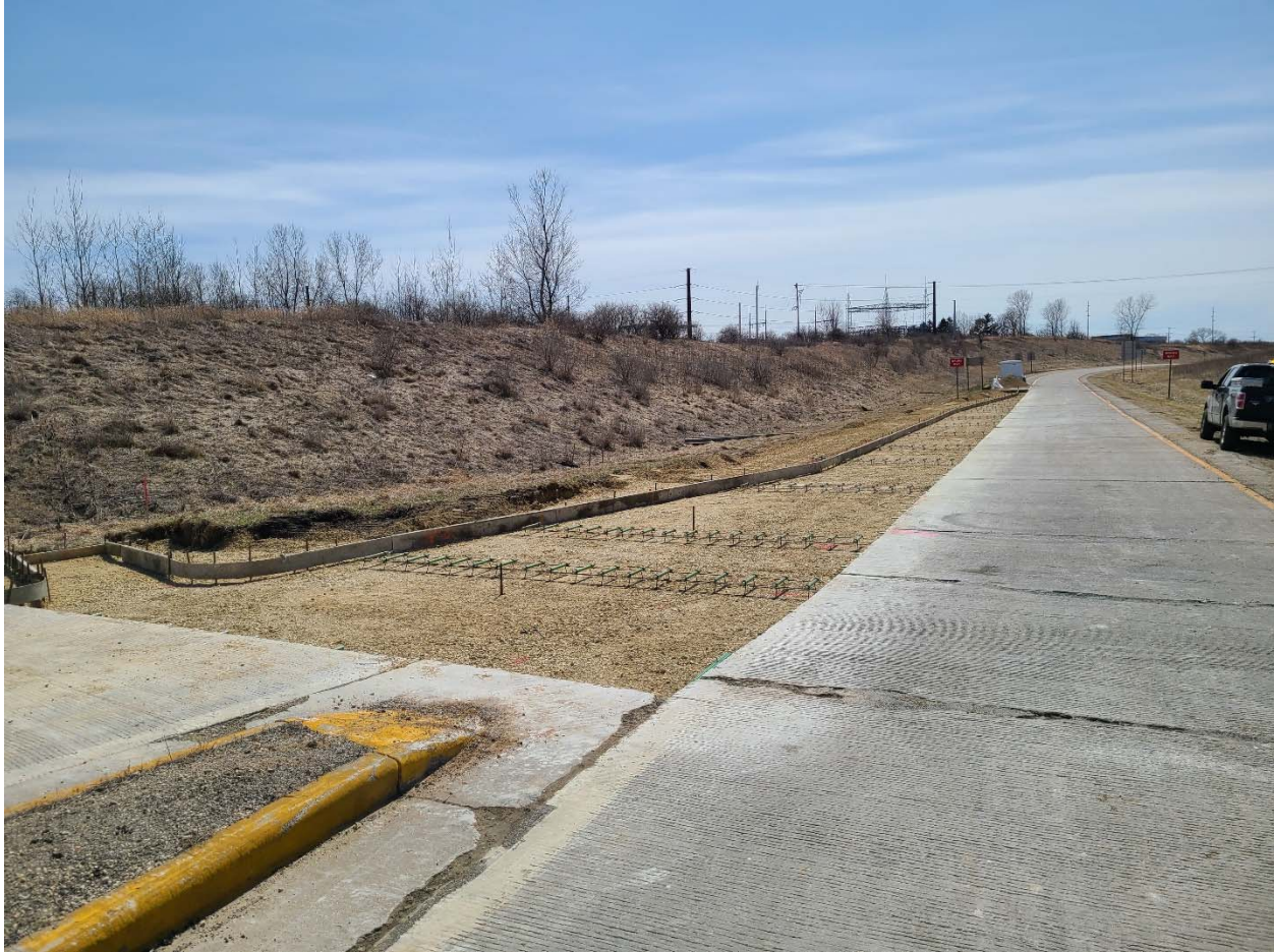
Figure 1: USH 18/151 EB Off Ramp Completed Concrete Pavement and Asphalt Shoulder.
