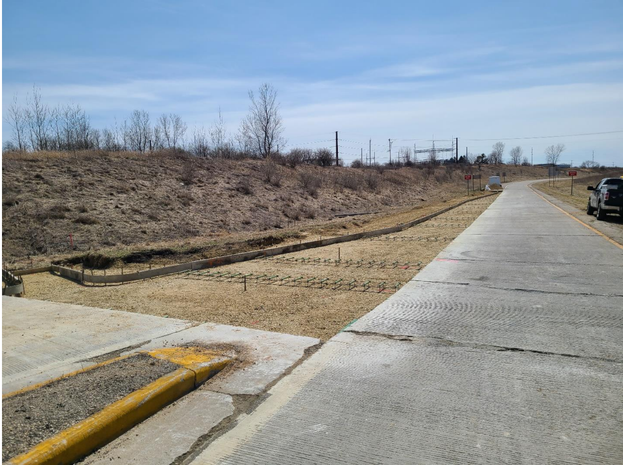
Figure 1: USH 18/151 EB Off Ramp to CTH PB Concrete Pavement Widening Prep.
