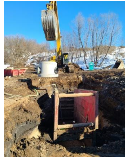
Figure 1: Setting Gravity Sewer Manhole at the Badger Mill Creek Horseshoe
